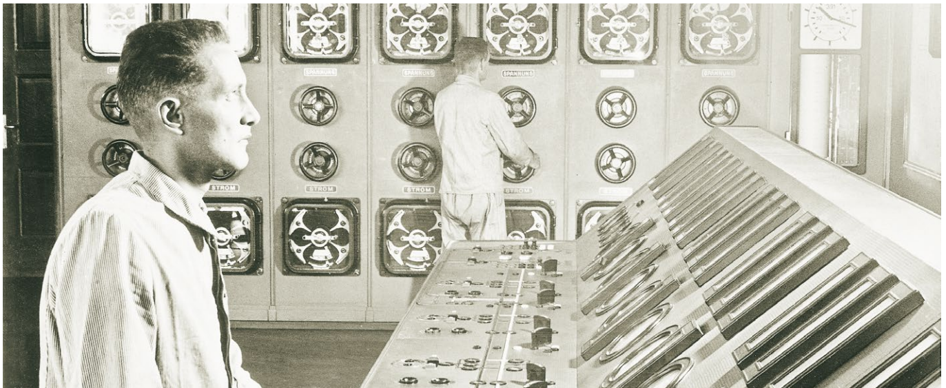
Control room, Gösgen power plant. Built in 1917, this power plant is now one of the largest run-of-river plants along the Aare with an annual production of around 300 million kWh. The people pictured were already insured by PKE's predecessor, Pensionskasse Schweizerischer Elektrizitätswerke. (Photo taken around 1921, Alpiq Ltd.)
